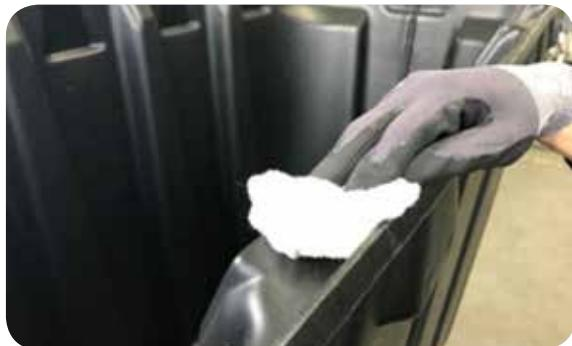
Clean the edge of the tank with a dry cloth, removing any grease if necessary
