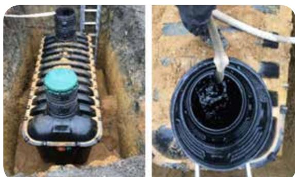
Self-levelling sand backfill at a constant level
