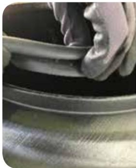
Put the manhole seal into place
