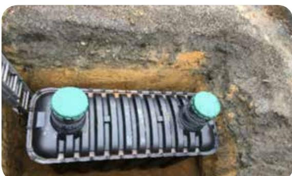
Position the tank in the bottom of the excavation
