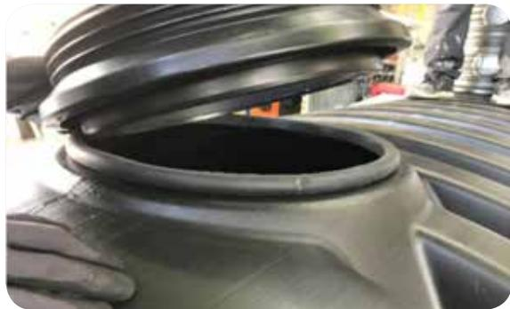
Slot the manhole into position
